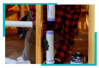
**d)** Plumbing issues related to riser clamp usage. A commonly misunderstood technology is the riser clamp, which is used to secure the pipe at the floor and prevent the riser from falling. Issues can involve the number of riser clamps needed, incorporating riser clamps into the expansion or contraction of piping, and properly installing riser clamps. These are all factors we've seen that can lead to systemic plumbing issues related to the riser clamp.
