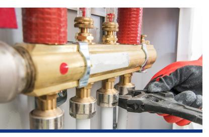
Another example is PEX piping. When it was first introduced, the product worked relatively well for cold water lines and it was thought that it would work similarly well for hot water lines. However, problems began when they started using the product in recirculating hot water lines. The PEX piping became embrittled, cracked, and eventually leaked. Entire systems had to be replaced. Because of these issues, new PEX products have been made that are built to handle these situations.
